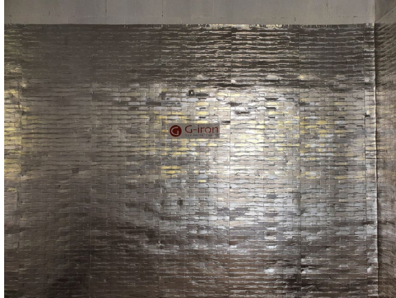
Picture 13 - G-iron ArmoFlex® installation completed
