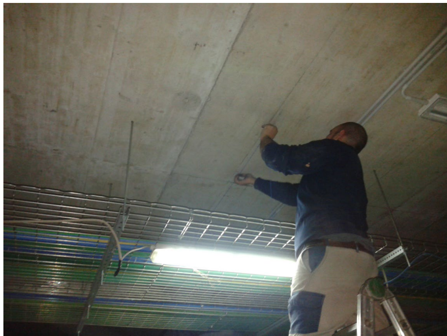
Picture 4: Outlining the surface to be shielded with a chalk line
