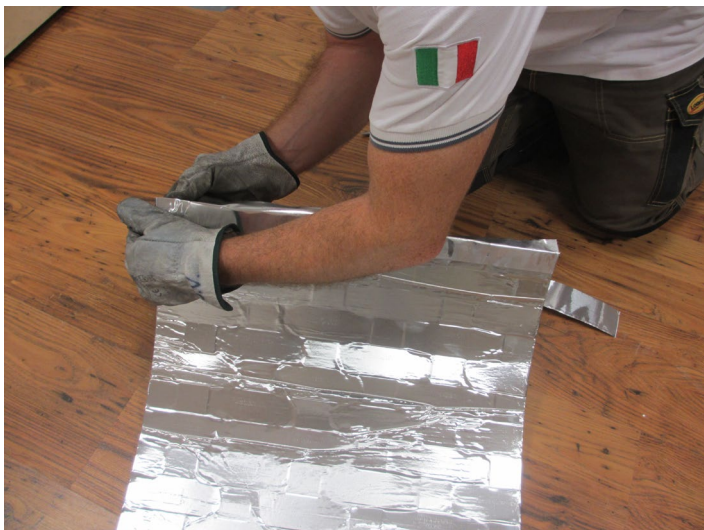
Pictures 7 & 8: Taping the cuts of G-iron ArmoFlex®
