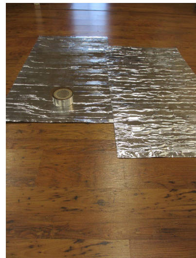
Pictures 7 & 8: Taping the cuts of G-iron ArmoFlex®
