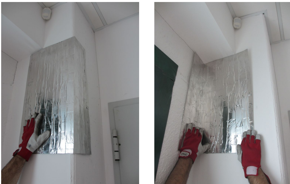
Pictures 11 & 12 – Vertical angular elements
