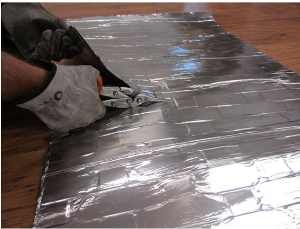
Pictures 4 & 5: Cutting G-iron ArmoFlex® with industrial snips
