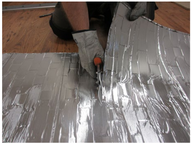
Pictures 4 & 5: Cutting G-iron ArmoFlex® with industrial snips
