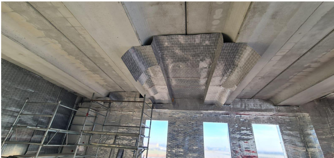
Fig. 3 installation on walls (ArmoFlex) and ceiling (SuperFlex)
