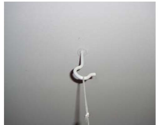
Screw Hook into Drywall Anchors
